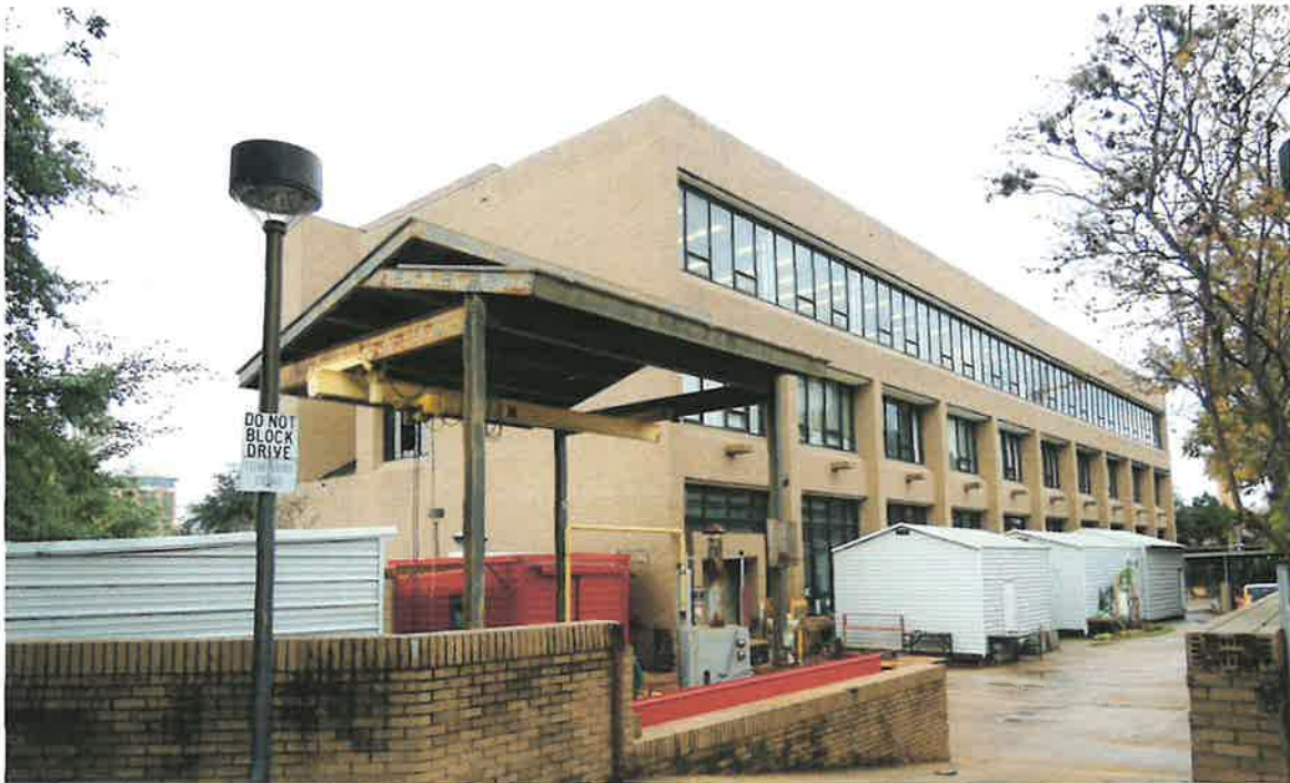
Before 6, Surrounding Structures, Photo taken at ground level North End
