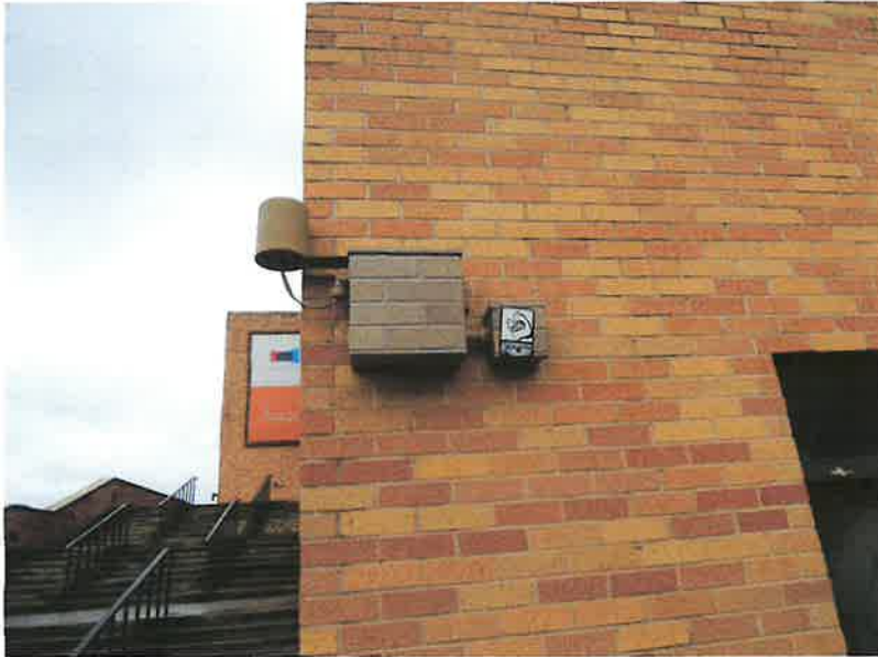
a. Modern electricity, intrusive restoration. w/ preserving the original artistic facade
